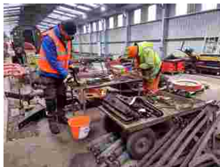
Volunteers team leader Richard Dovey and Ralph Sanders cleaning Pullman kitchen car no. 99361 brake linkage components in preparation for inspection and re-painting
